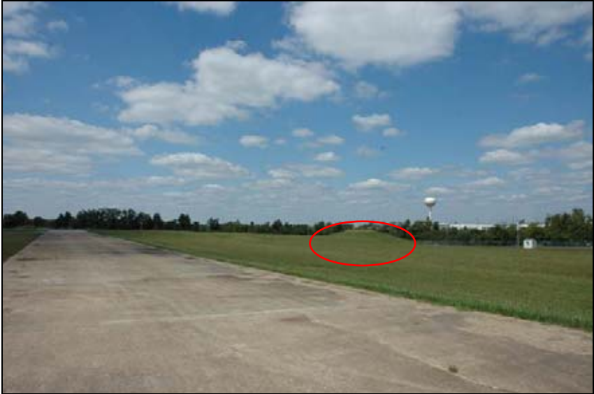
Figure 1 (North End: Berm)
