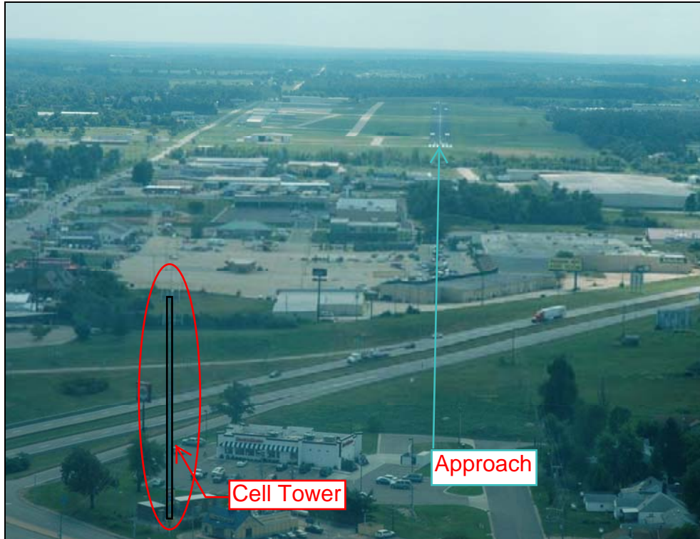
Figure 5 (North End: Approach)
